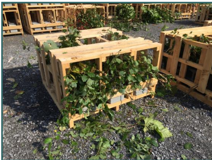
Short-plank vertical structures are created to provide habitat for large game-fish in the lake.
